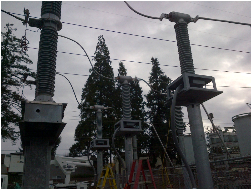
Figure 7. Electrical Phenomena Cluster (EPC), which can optically measure current, voltage, and temperature. No active electronics for E1 vulnerability instead optical cable transmits light signal to and from the control house. No conductive cabling required.
